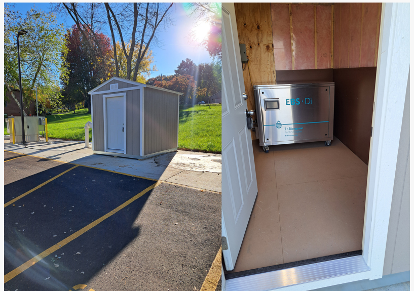
Additional EBS-Di Unit Installation at Secondary Lift Station Structure
