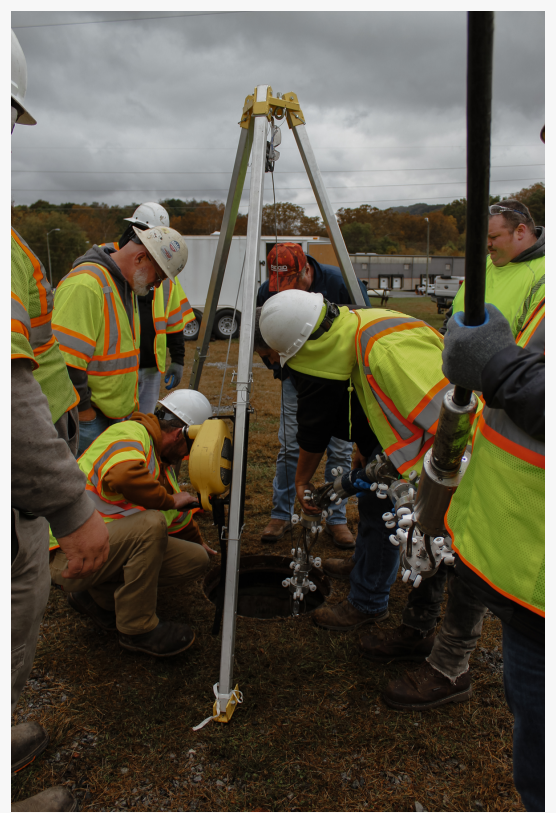
Deployment of the UV Curing Lighttrain
