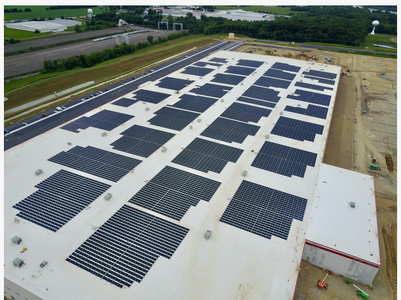
Commercial Installation with over 10,500 solar panels
