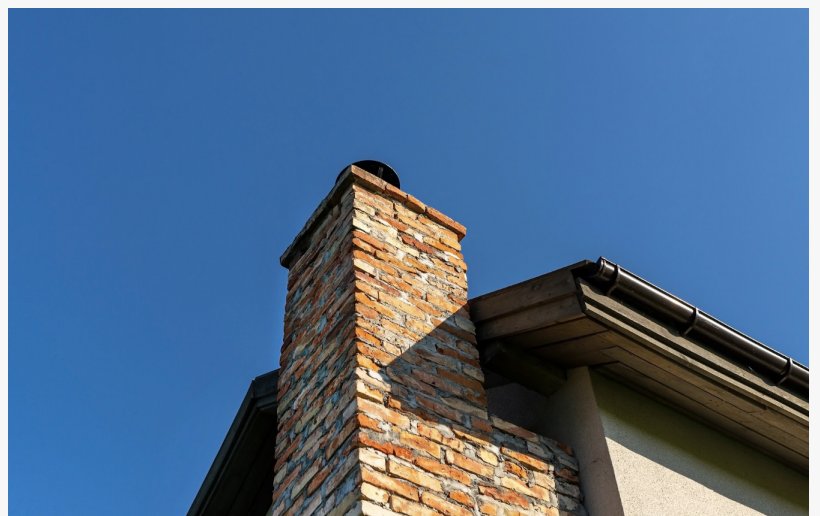
Image of a brick chimney from below.
