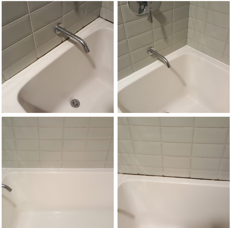
Before and After bathroom shower/tub grouting repair
