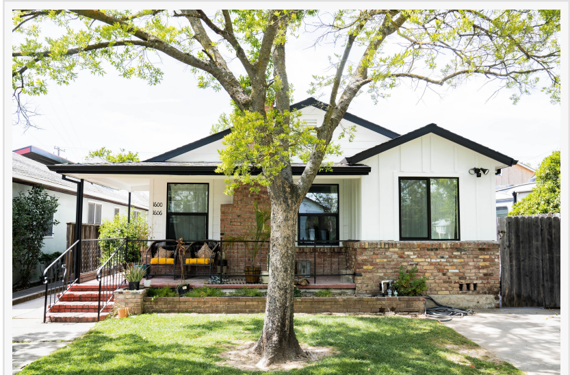
bay Area Siding Contractor
