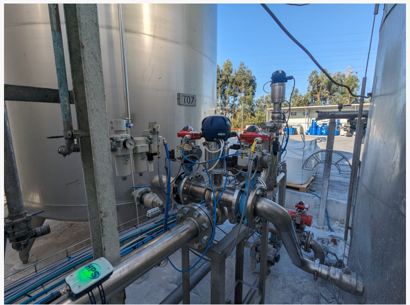
HPS Advanced Liquid Product Recovery Technology
