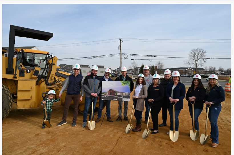
Ducklings Early Learning Center Whitehall Groundbreaking
