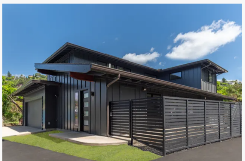
A new home built by H-1 Construction
