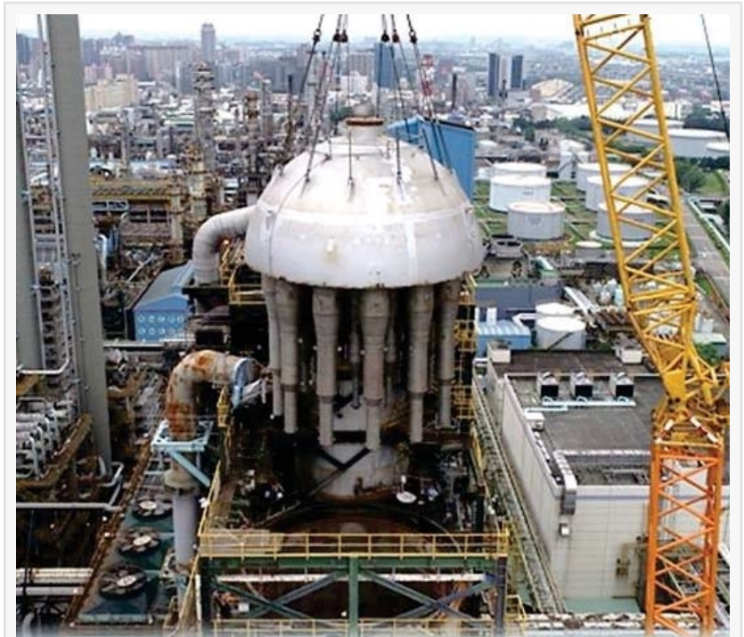
Ducon Refinery FCC Cyclone Installation
