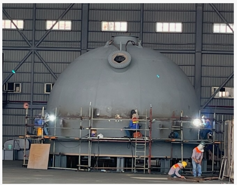
Regenerator Vessel head fabrication in Ducon Shop
