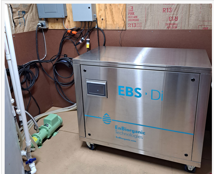
Installation of EBS-DI in North Utica IL
