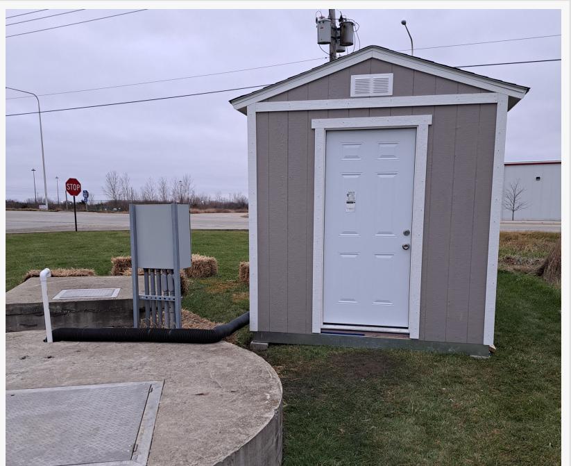
Lift Station Installation Site
