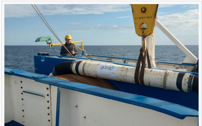
Image of one of the three SMART cable instrumented repeaters being deployed.
