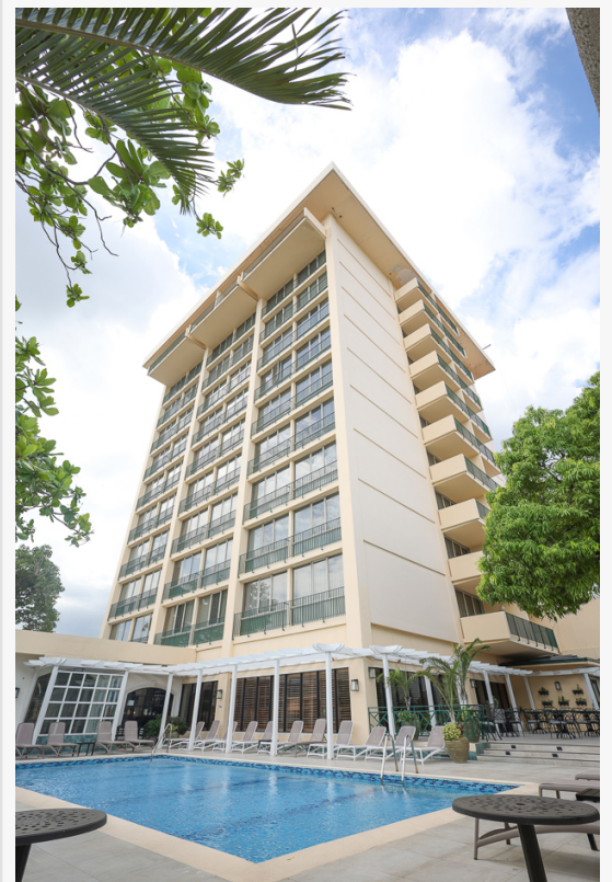
Exterior of the newly-renovated Courtleigh Hotel and Suites, Jamaica
