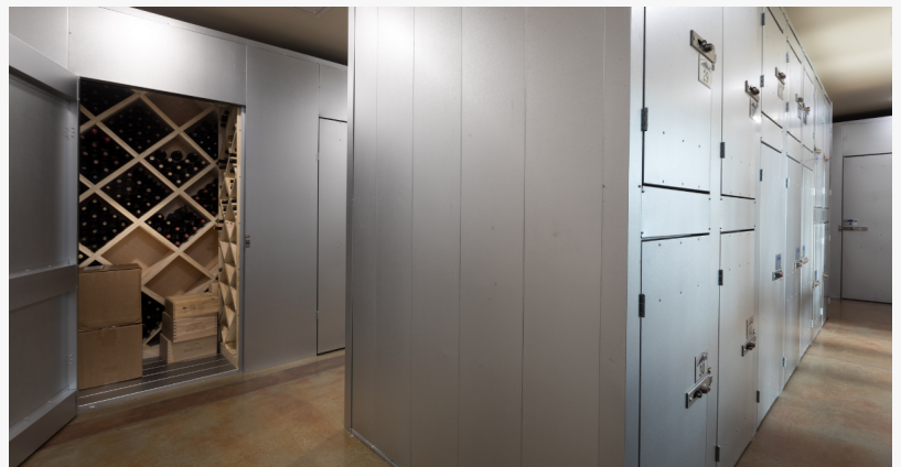
Premium Wine Storage Vaults
