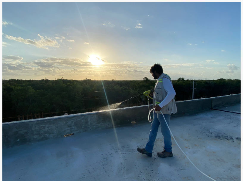
TechCrete 2500 application in Tren Maya Project, Mexico
