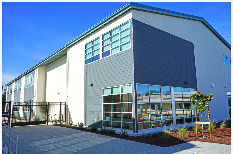
Newly Constructed Two Story Building - Ravenswood Middle School
