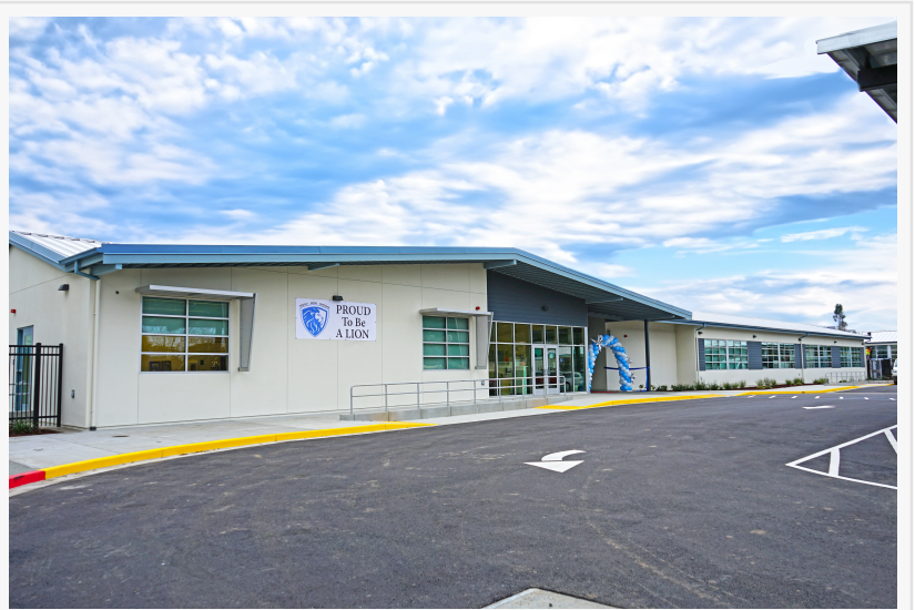
New Entry Building - Ravenswood Middle School
