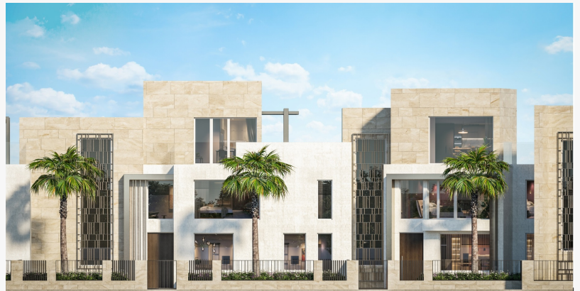
Liv Waterside Villas in Dubai Marina
