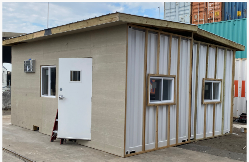
Unique community center constructed from two seamlessly welded shipping containers
