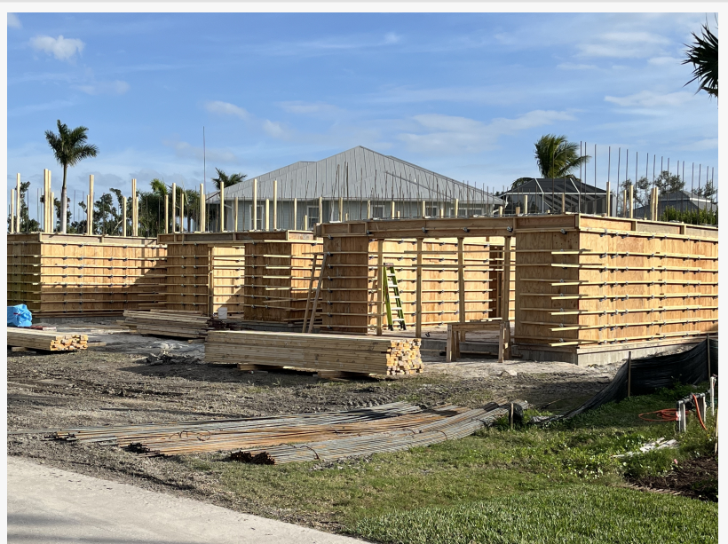
Formwork for Solid Concrete Foundation Walls
