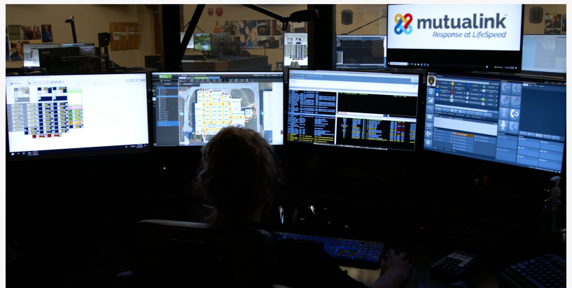
Mutualink System being used in Smith County 911 Dispatch Center
