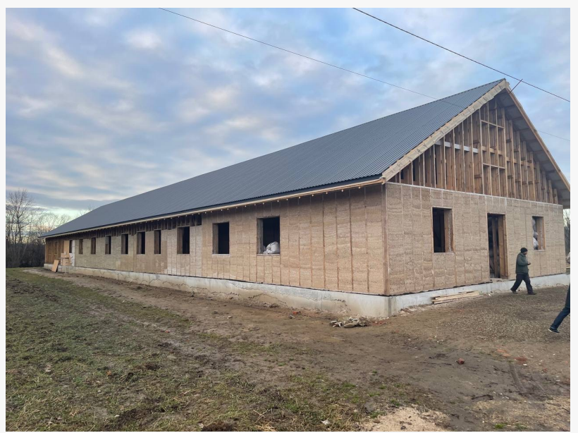
Hempcrete housing in Lviv, western Ukraine, sequesters 1,000 tonnes of CO 2 e captured from the air by hemp plants
