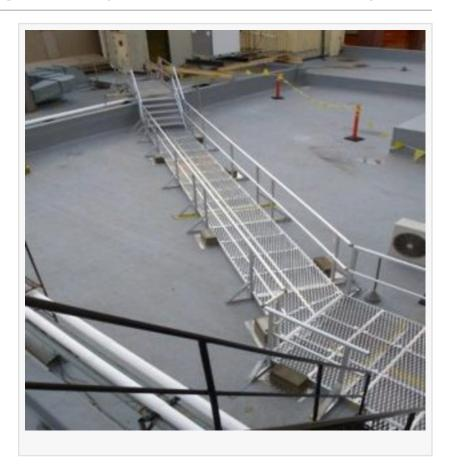
Rooftop walkway systems are engineered to protect the roof membrane from damage due to foot traffic and ensure that individuals can safely access necessary areas for inspection and maintenance tasks. This initiative not only extends the lifespan of roofing materials but also
