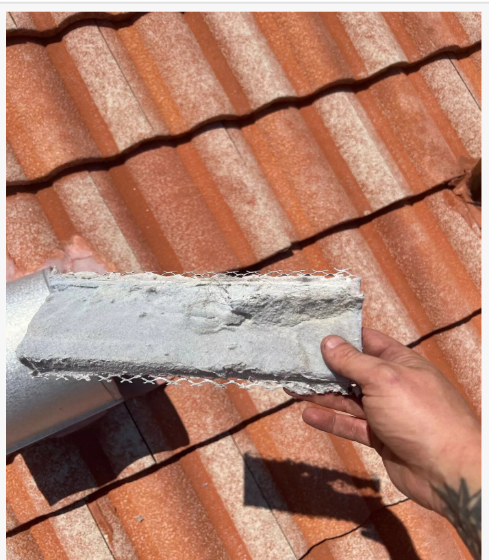
Air Duct Cleaning - Clean Quality Air
