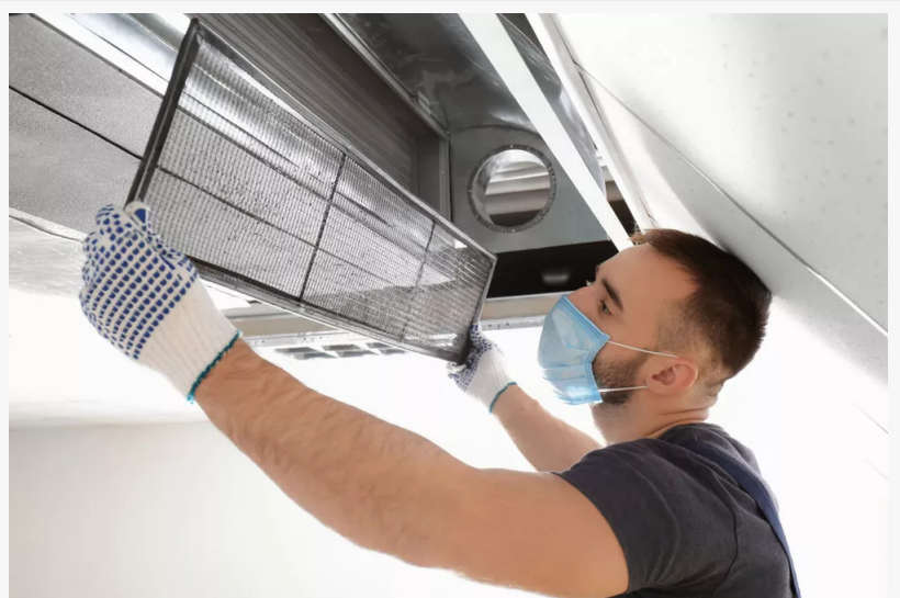
Air Duct Cleaning Services in Port St Lucie
