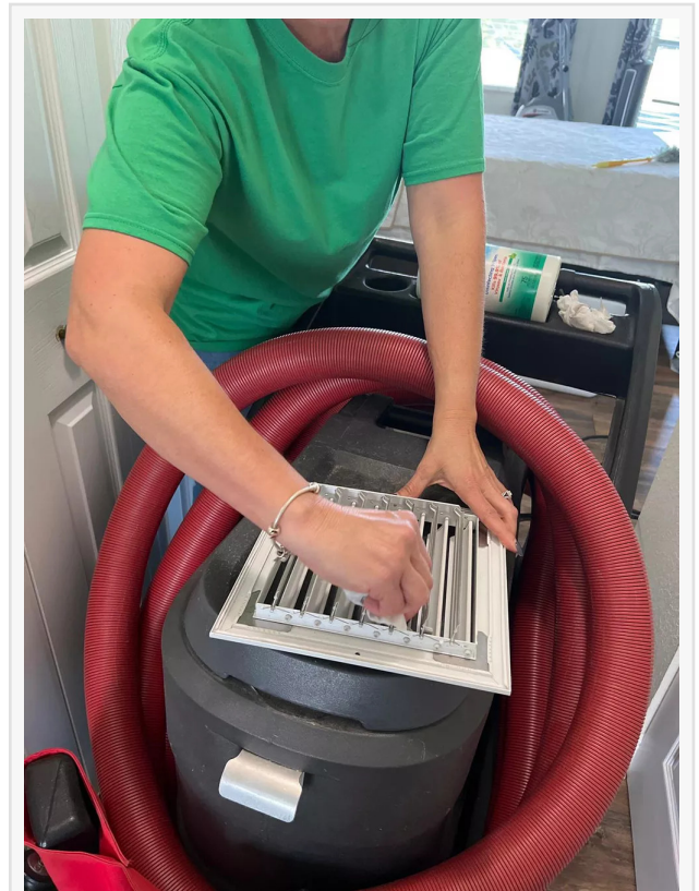
Air Vent Cleaning
