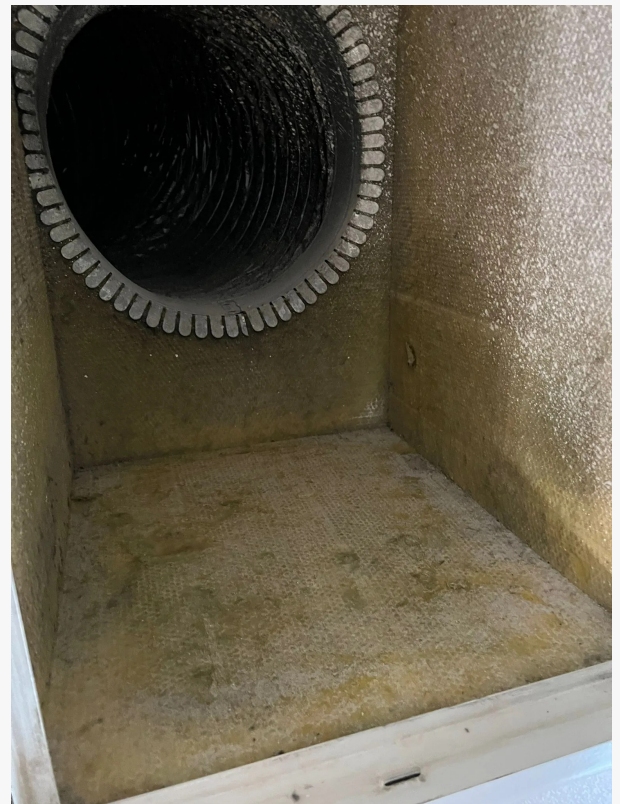
Air Duct Cleaning
