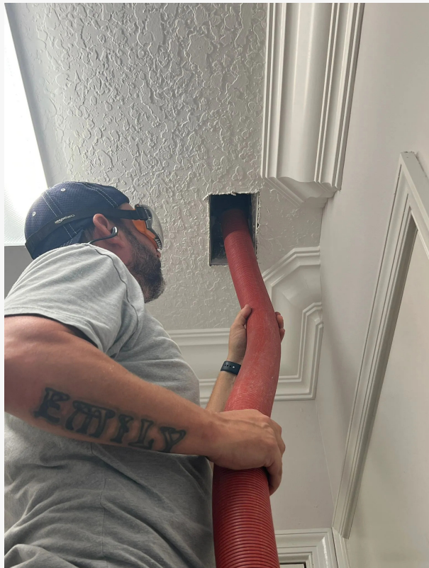
Regular Duct Cleaning
