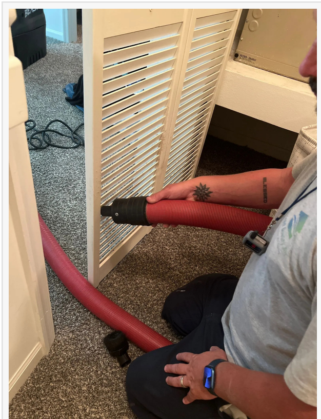
Air Duct Cleaning PSL
