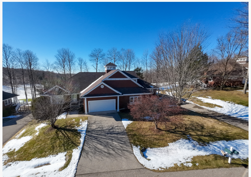
Aerial view of 620 Crooked Tree Drive
