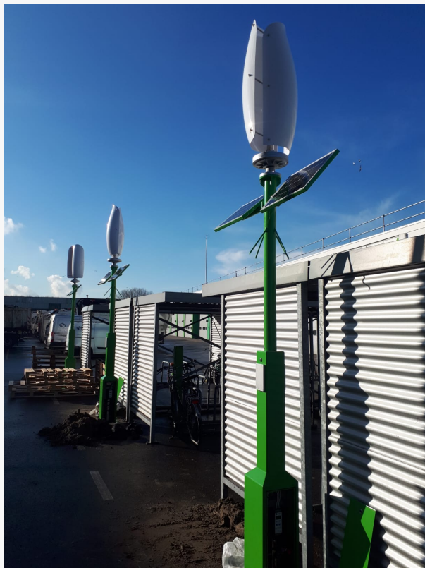
Wind and Solar E-bike Charging Poles
