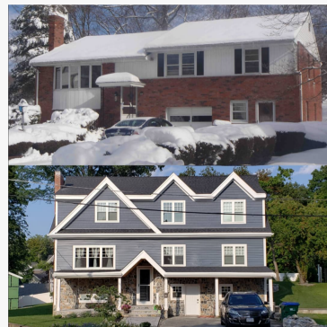
Home addition, 2nd story addition
