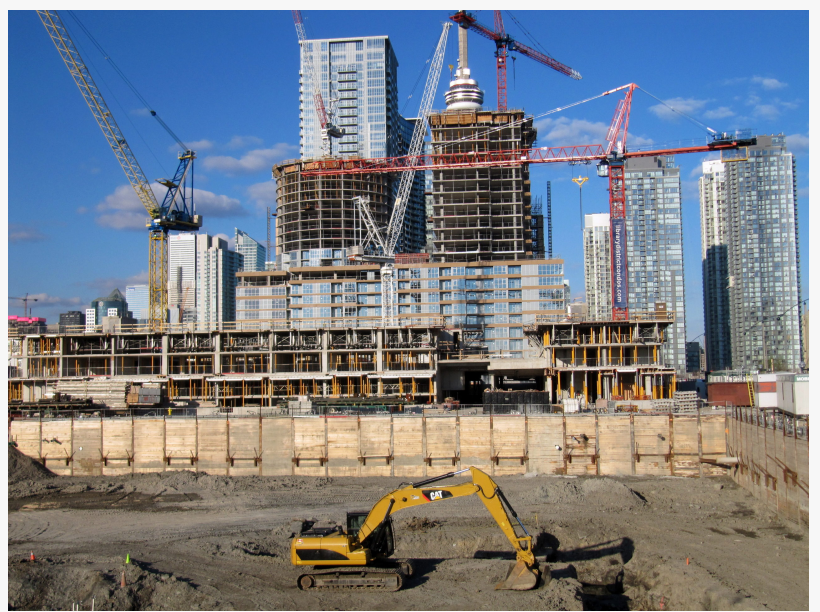
Construction site view
