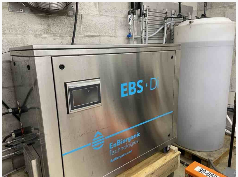
EBS-Di Installation at SSTA, 2nd Liftstation
