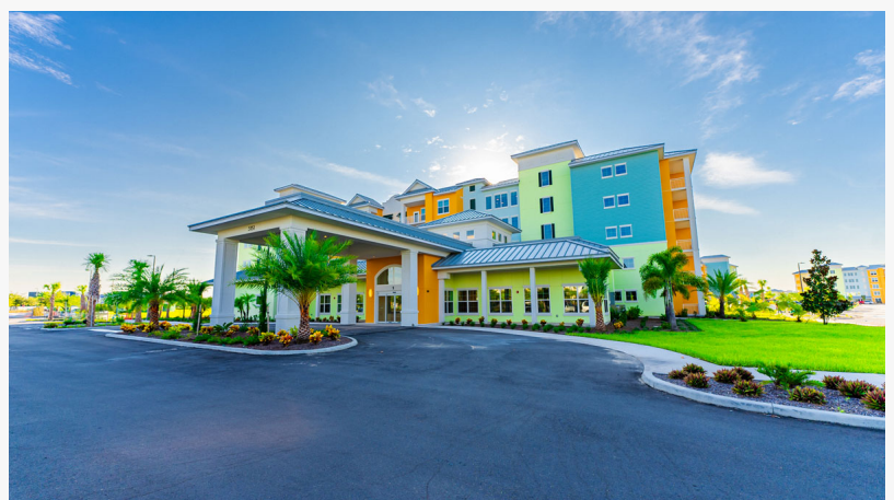
Building 1 & Amenity Center
