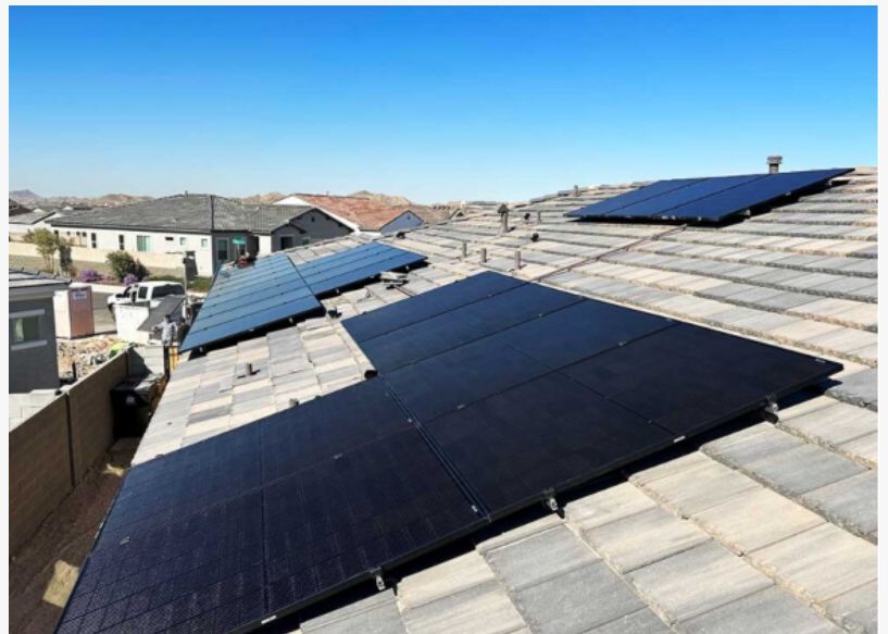
Arizona Solar Wave Residential Solar
