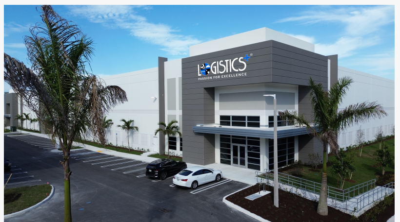
Logistics Plus Miami, FL Warehouse #2
