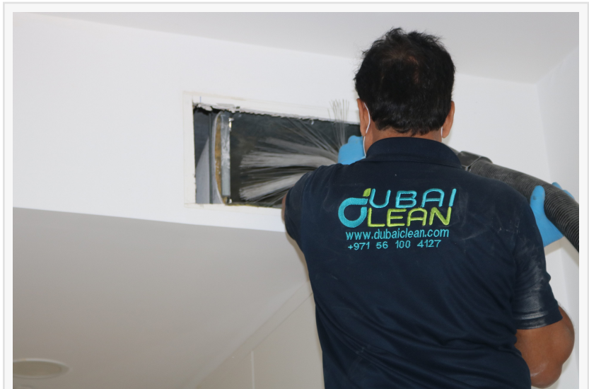
AC Duct Deep Cleaning Services in Dubai by DubaiClean
