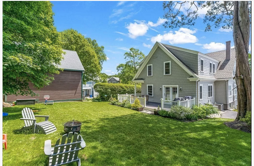
A rear home addition
