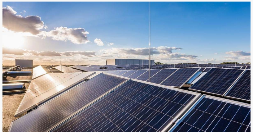
Common photovoltaic project base, photovoltaic panel installation.
