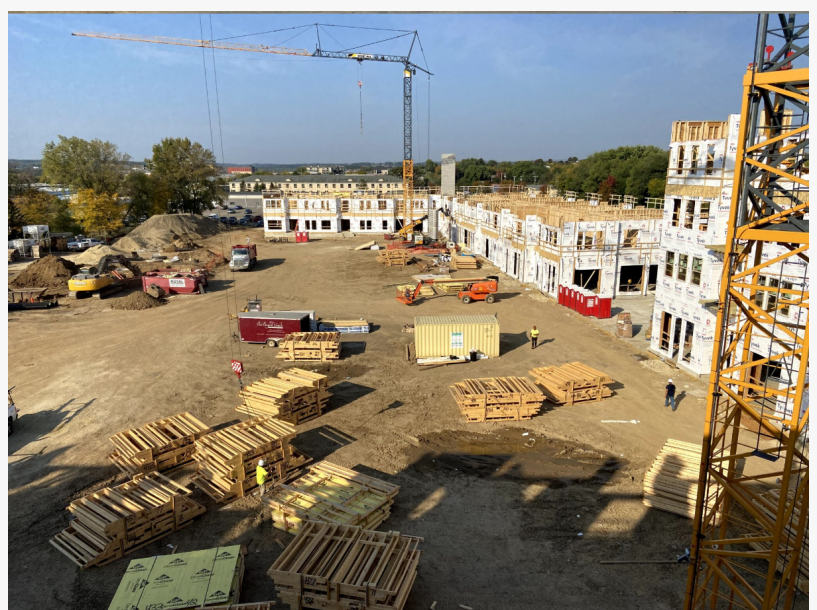
DC Materials LLC. Construction Site
