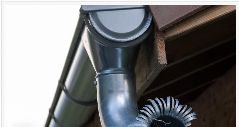
Gutters on the side of a house.
