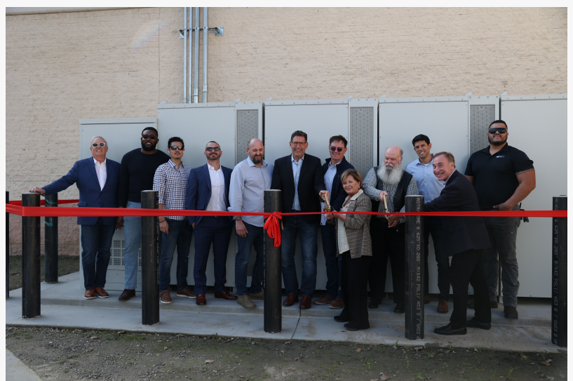
Blue Sky Utility executives, mall management and local elected officials prepare to cut the ribbon at the battery energy storage site at Hanford Mall in Hanford, Calif.
