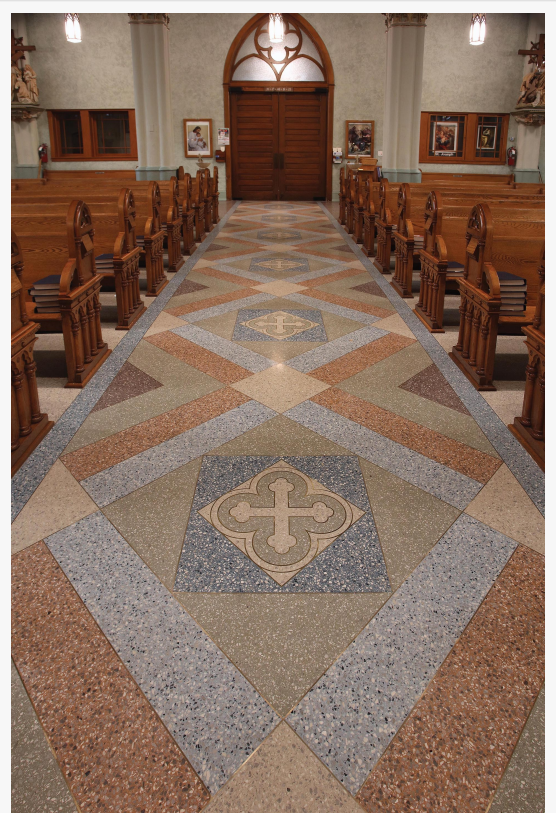
HAND-CRAFTED terrazzo was poured in place in the 1902 sanctuary.
