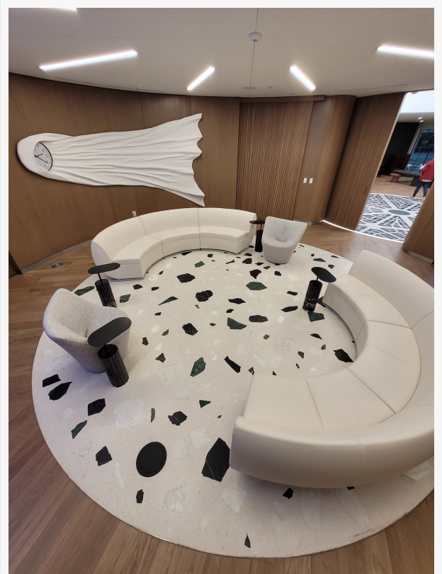
PALLADIANA TERRAZZO in Rock Ventures lobby incorporates large marble slabs in an epoxy matrix. John D'Angelo Photo
