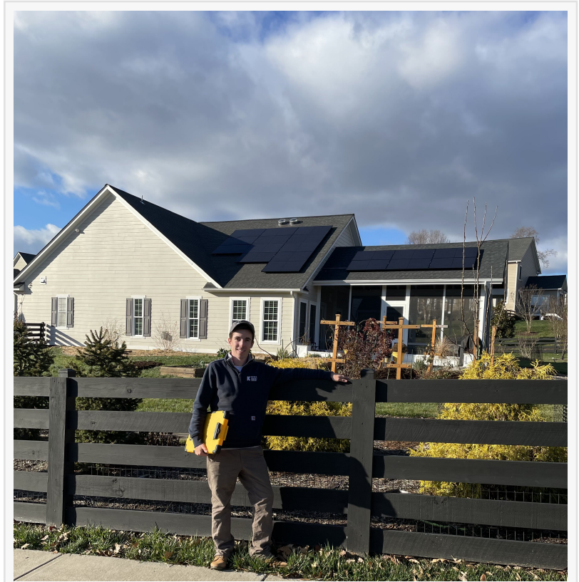
Kilo Hollow Energy rooftop solar array in Charlottesville, VA.
