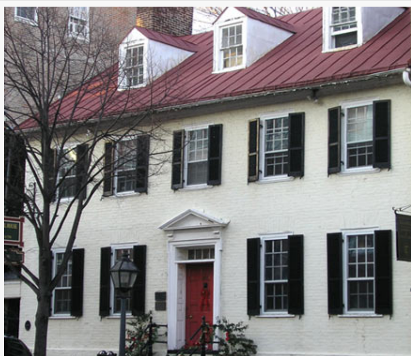
Replacement Windows Installations
