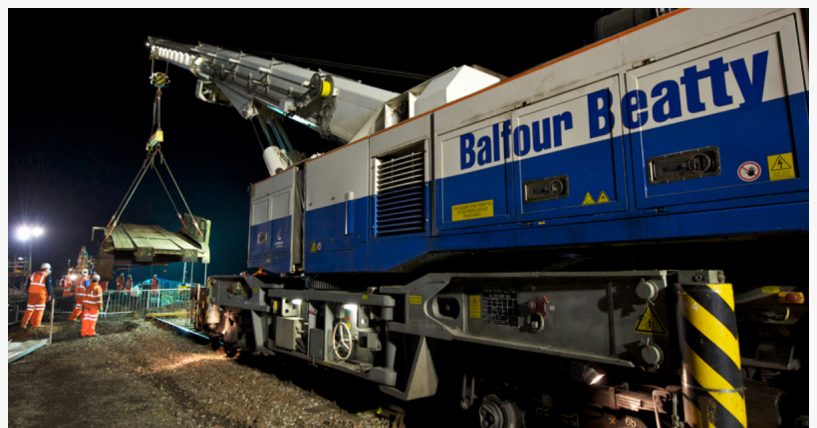
Balfour Beatty employees implement work at project site
