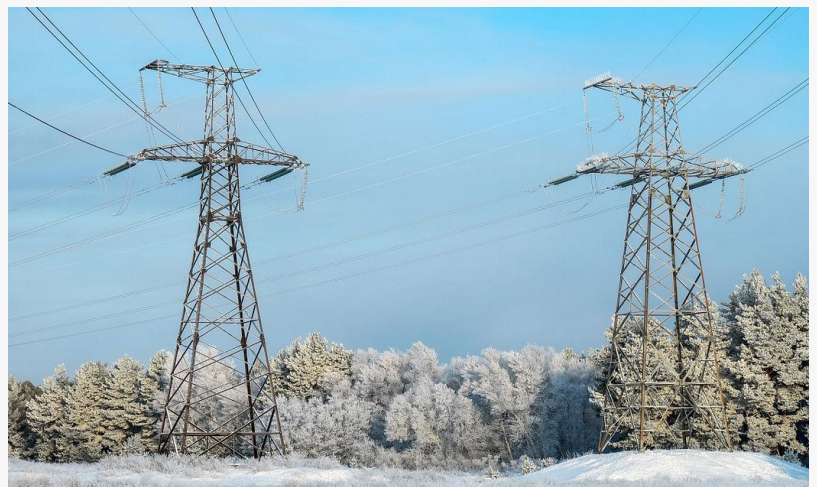
Alpine overhead lines in the north of Scotland
