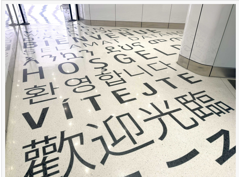
TERRAZZO installation in O'Hare Airport's new terminal A greets travelers in 29 languages. Photos by Joe Aldolino, Clayton Menconi
