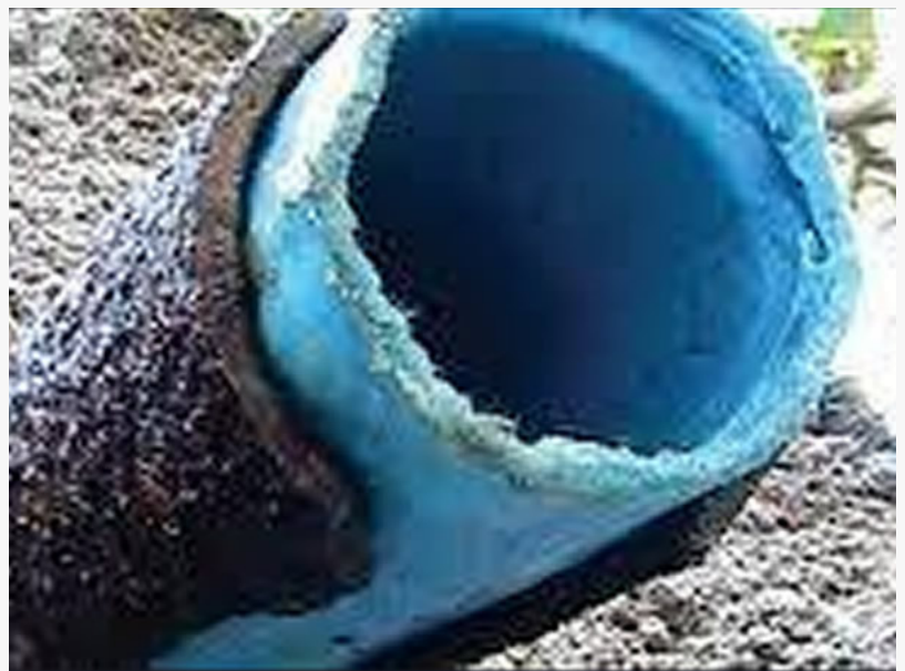
Lined Sewer Pipe Repair in Miami
