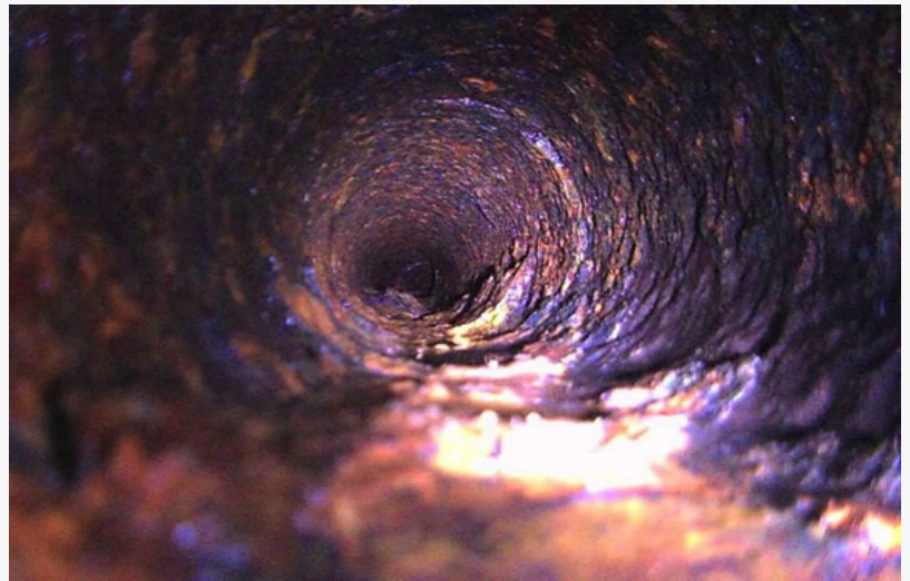
Sewer Pipe Repair - Miami Florida
