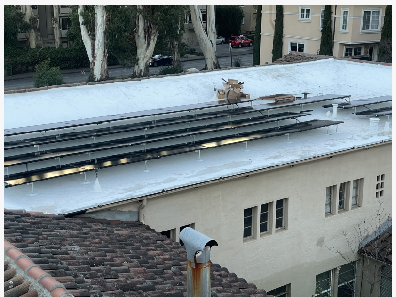
NLCC Solar Installation During Construction
