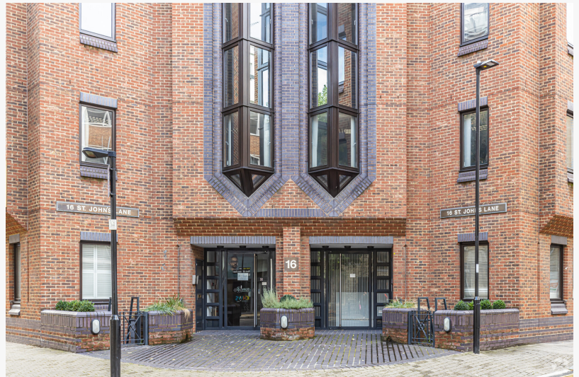
Maintech Europe Ltd Headquarters
