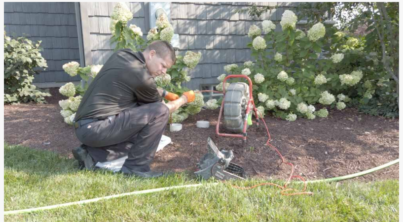
Plumbing and Drains Clean
