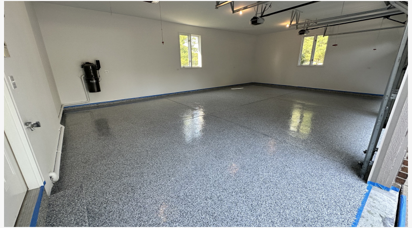
garage floor epoxy coat
