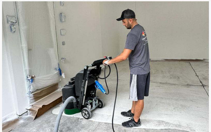
Concrete Preparations Process
