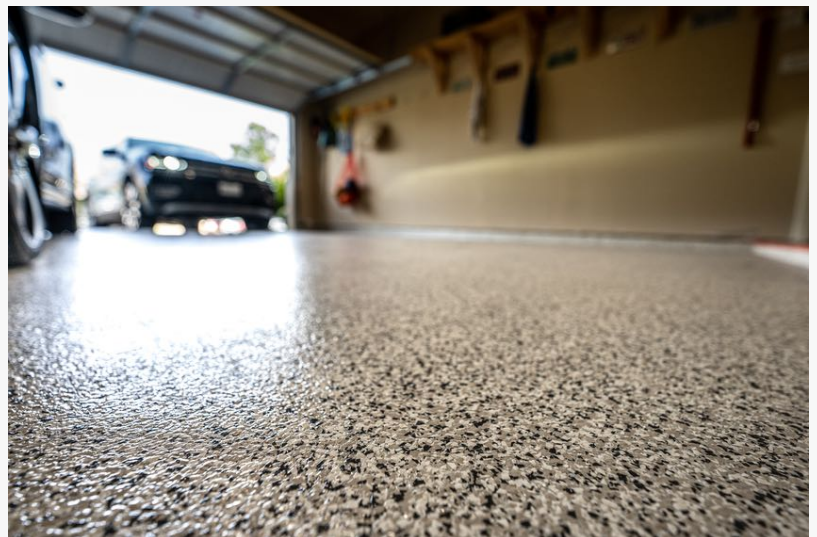
garage floor just coated epoxy
