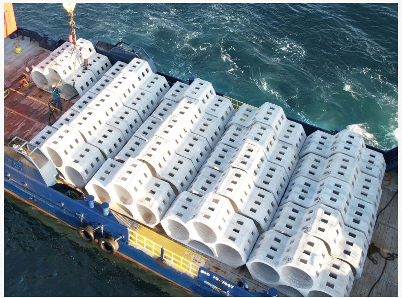
A total of 25 SEAHIVE® units for marine habitat were efficiently deployed off the coast of Destin-Fort Walton Beach within a single day.
